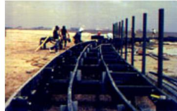
PCRP has UV and plasticizer additives in its mix and replaces traditional creosoted and CCA pressure treated timbers. It has many advantages: it is environmentally friendly; it is resistant to marine borers; it has a higher flash point than traditional timbers; it has an infrequent maintenance need; and it does not split, delaminate, rot, corrode or spall. It is also cost effective on a life- cycle basis even when considering the higher cost of the material.
