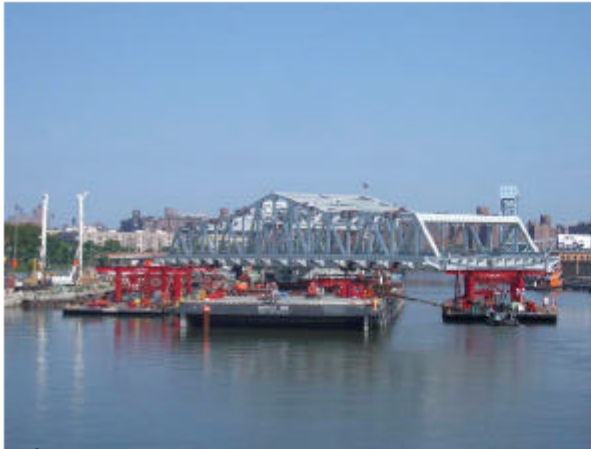
3 rd Avenue Bridge – New York City
