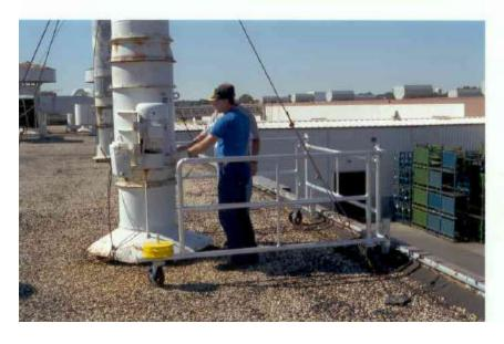
Mobile Parapet Barrier being used to safeguard workers at roof edge.
