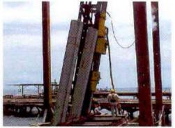
Driving pile: sensors are inside red square, connected by cable to PAL-R.
