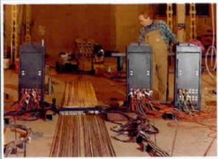
Most projects require the an even lift to avoid cracking or stressing the structure. Using Liftplate's patented synch24 control system, all lifting points are synchronized with a high degree of accuracy.
