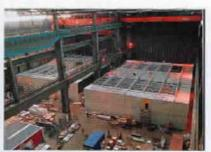
The construction of modules takes place Entire plants can be assembled indoors for maximal control. Example: A 50,000 sqf facility for Eli Lilly & Co.
