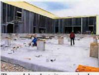
The modular plant sits on a simple foundation that has been prepared in advance by the Client.
