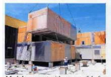
Modules are set with a pace of 4-6 per day. In a few days to a week or two the from a conventionally built plant. entire building is installed at the final site.
