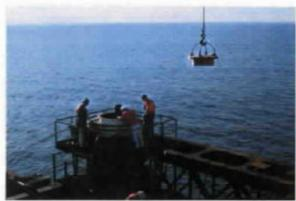
3. When the caisson was dry, a smaller pipe was inserted into the caisson and a diver was lifted by mancage into the pipe. When he reached the top of the diffuser, he opened the manhole cover that separated the diffuser from the outfall lunnel below. A crane lifted the cover away from the manhole.
