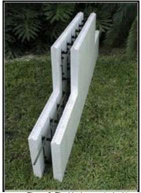
Figure 2. The blocks are stacked together
