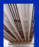
In addition to internal prestressing, each Structure B beam was externally posttensioned with (4)-40mm (1.6 in.) diameter CFRP cables.
