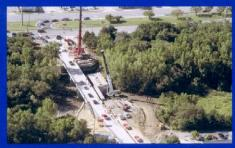
Two 500-ton mobile cranes were used to set the doubletee beams for Structure B.
