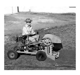
The DWP trencher is used to prepare for the installation of a water line.
