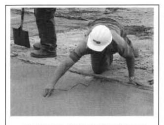
Paving contractor embeds intelliRock sensor in freshly poured section of pavement
