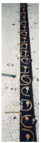
Tie Steel Projecting from Panels Over Supports, Anchored Around Studs
