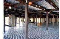
Left: corrugated pan deck is installed ready for concrete.
