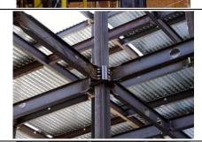
Left: completed stable unbolted moment collar connection which forms a Node.
