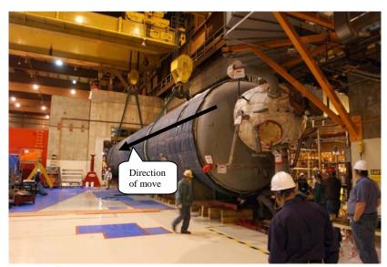
Sliding new vessel into place to 2" clearance
