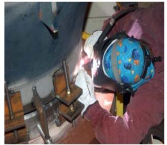
Welding new vessel to 48" piping
