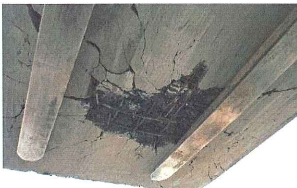
Bottom of Slab
