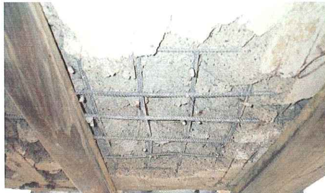
Bottom of Slab
