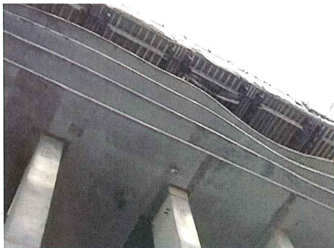
MCO® used in deck forms in a major high-rise building
