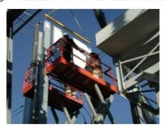
Fig 6. Installation of Pre-Fabricated Panels
