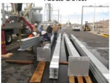
Fig 4. Installation of Pre-Fabricated Vertical Columns
