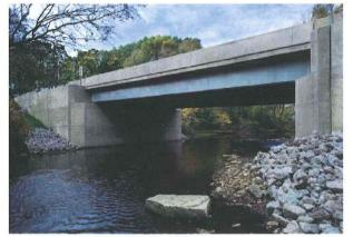
HIGH ROAD BRIDGE, LOCKPORT TOWNSHIP, ILLINOIS This bridge consisted of six (6) HCB's 58"-4" long x 42" tall with a conventionally formed cast-in-place concrete deck.
