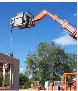
Because the Mix-N-Place™ mixer and delivery system is taken to the tubs, instead of the tubs to the mixing site, the tubs never leave the scaffolding. This means you don't have to try to set the tubs back on the scaffolding.
