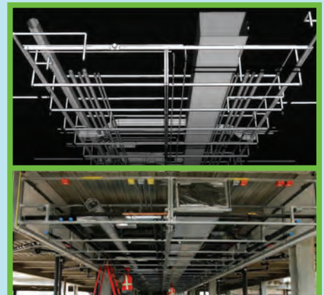
MEP corridor racks BIM model design and final MEP corridor racks installed
