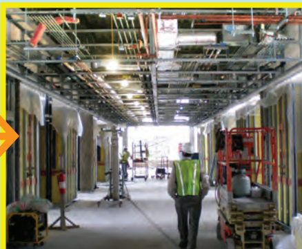
MEP corridor racks being installed
