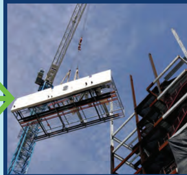
MEP corridor racks being lifted to the floors
