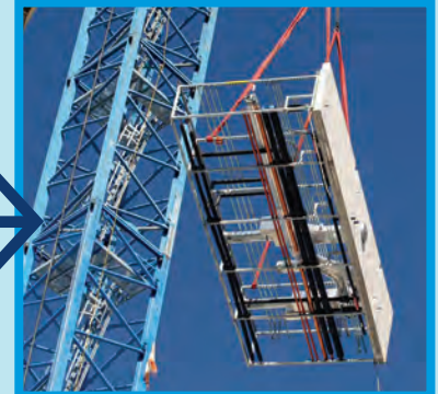
A tower crane lifting the MEP corridor racks
