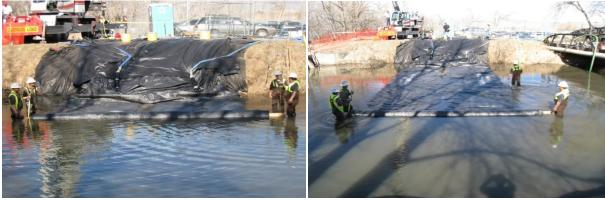
**Step 3:** Two identical pumps are hooked up to fill the internal tubes with **Step 4:** As the pumps fill the Dam, the Dam unrolls and is guided into place
