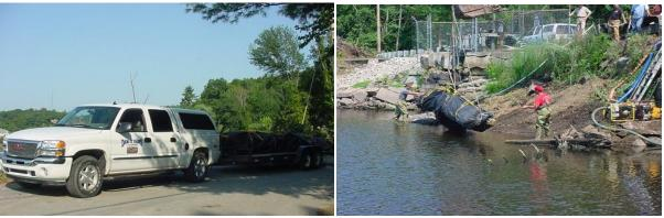
**Step 1:** The rolled-up Dam is delivered to the job site on a truck or trailer **Step 2:** The Dam is lifted from the trailer and placed at the shoreline
