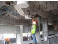
URS developed a first-of-its-kind air pressure system installed beneath the concrete shell.
