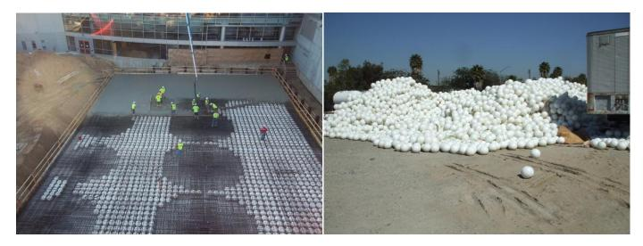
Concrete top pour at the LaBahn Arena in Madison, Wisconsin (top, left) Plastic Balls at a Precast Facility (top, right)
