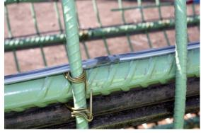
Digital thermal sensor on cable
