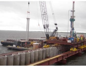
**Closer Pile and Grout Plum Template and Platform**
