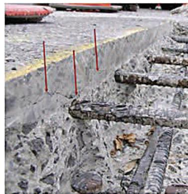
Example of bridge deck delamination
