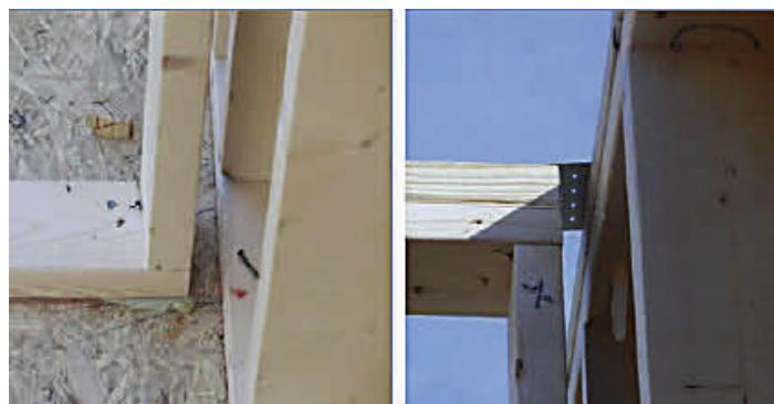
The interior wall framing is anchored to the top plate of the exterior with a flat plat connector.
