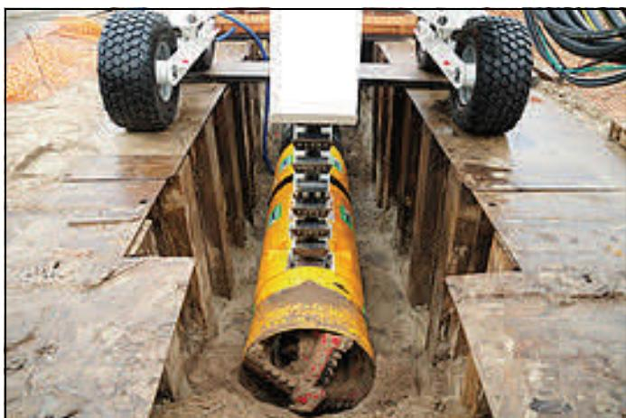
**Modular design:** A TBM that works underground and a trenching unit as a vertical connection between the TBM and the terrain surface.
